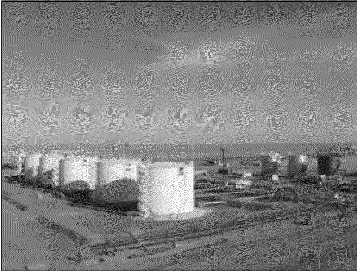
Oil and Condensate Storage Tanks at Opornaya
