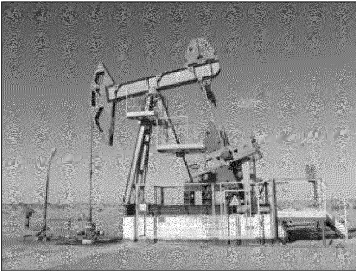
Borankol Oil Well Pumping Unit
